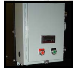
Standard auto-fill valve and interlocking control panel shown. Features built in, pre-wired controls.
